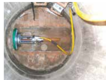
BURSTFIX 200 inside the manhole
