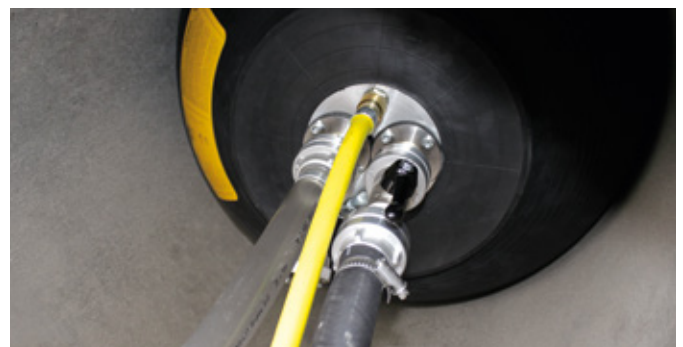
Water pressure testing
