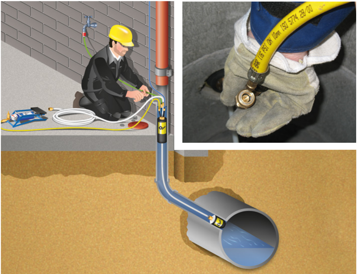
Water pressure test according to DIN EN 1610 with the Vetter test system for domestic pipe network
